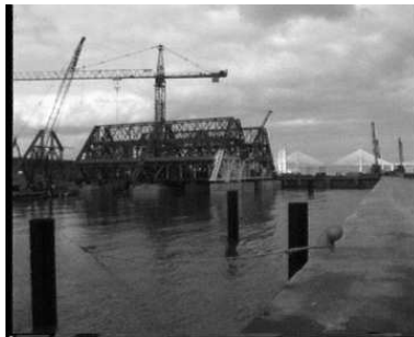
(a) Building under construction
